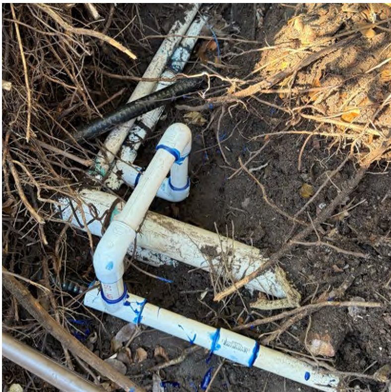
Lateral repair under oak tree along south side of Ayersworth
